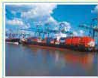
Deepened & Widened Channel
